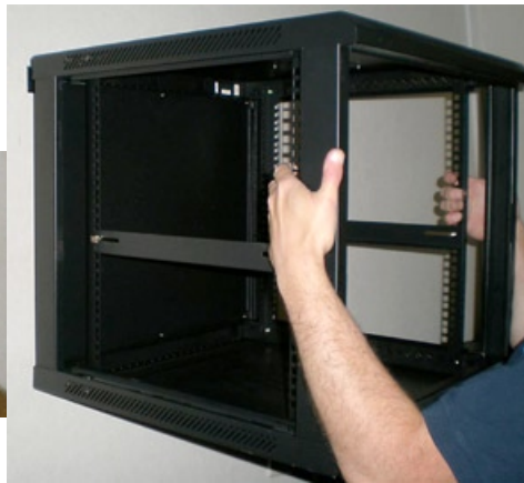
Easy mounting of the wall cabinet on the wall mount bracket
