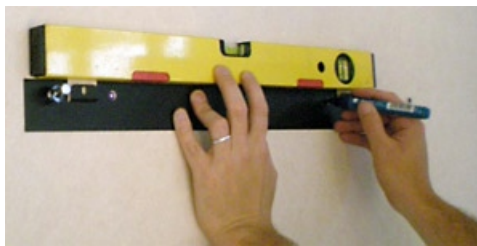
Install wall mount bracket
