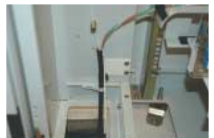
Loose Tube, High Fiber Count, cable entering at the left bottom side.
