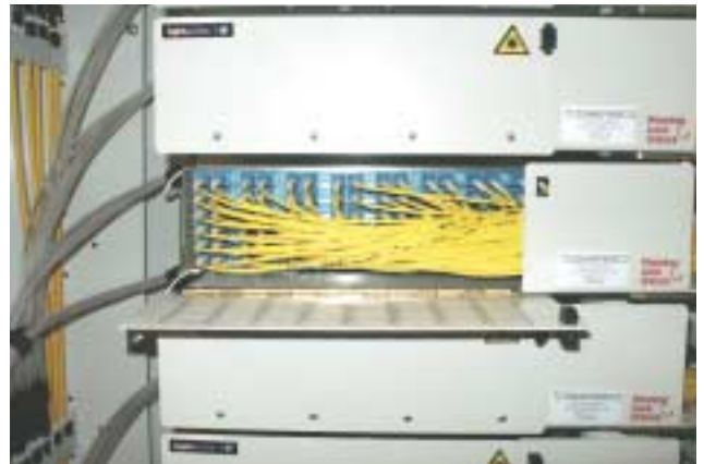
Open the cover plate for access to the patchfield.
