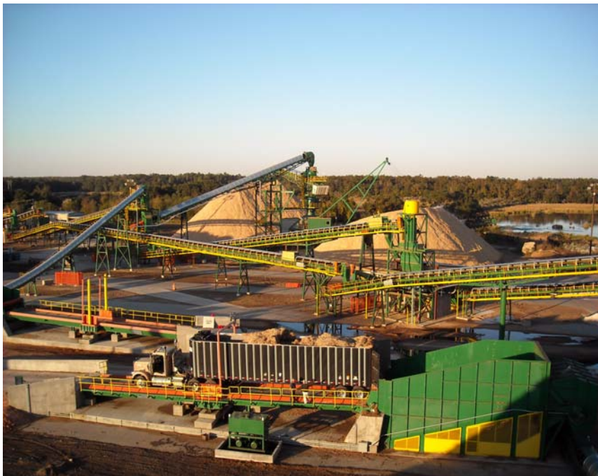
Fulghum Industries provides conveying systems and other heavy duty equipment for the woodyard in Valdosta.
