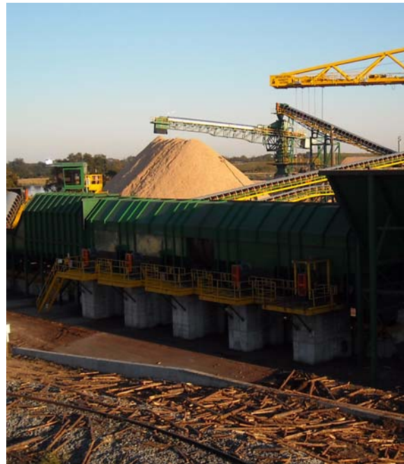
Rockwood stacker-reclaimer (center) at Packaging Corporation of America's Valdosta, GA facility.
